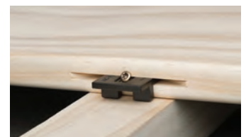
Local grooving, with a Lamello® type biscuit joiner or a router.
