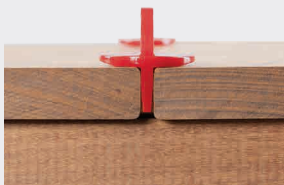
5.5.4.2.2 Spacing between decking boards
